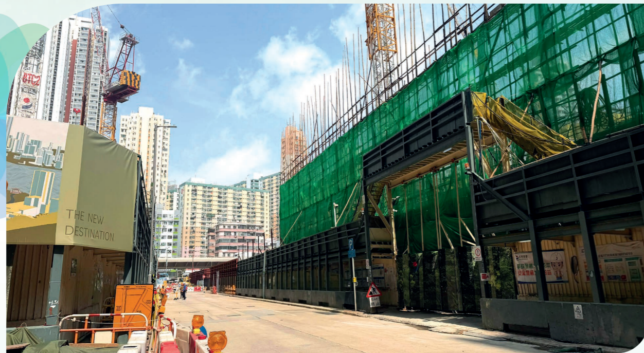
To Kwa Wan redevelopment project
