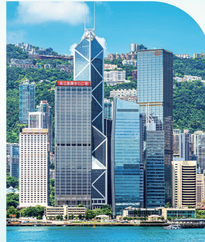
Overlooking Victoria Harbour, Cheung Kong Center II is set to become the new jewel in the crown that is the Central waterfront skyline.
