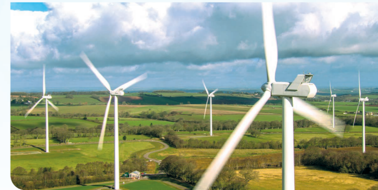
Den Brook Wind Farm generates enough renewable electricity to meet the annual energy needs of approximately 13,000 homes in the UK.
