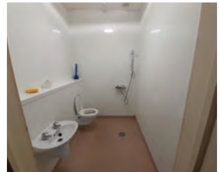
Fully accessible bathroom refurbished to doc M building regulations.
