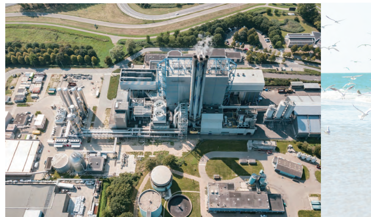
AVR's Waste-to-Energy Plant in Duiven
