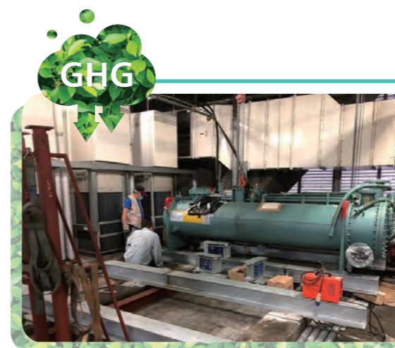
Replacement of chiller at Cheung Kong Center
