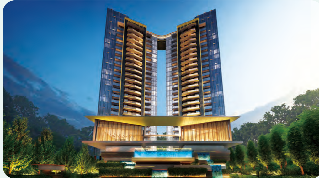
A sky-bridge garden connecting the twin towers allows residents to dine and relax in privacy (Artist’s impression)
